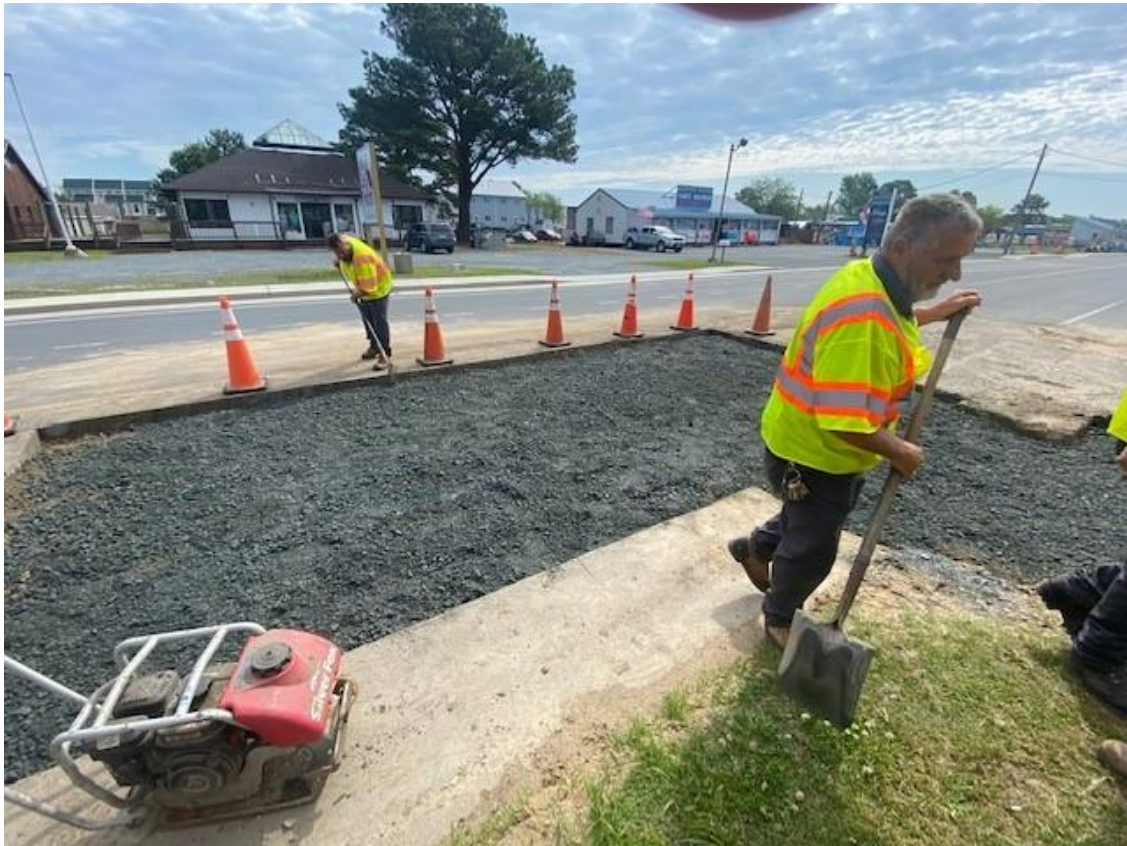
Placing and compacting new base material
