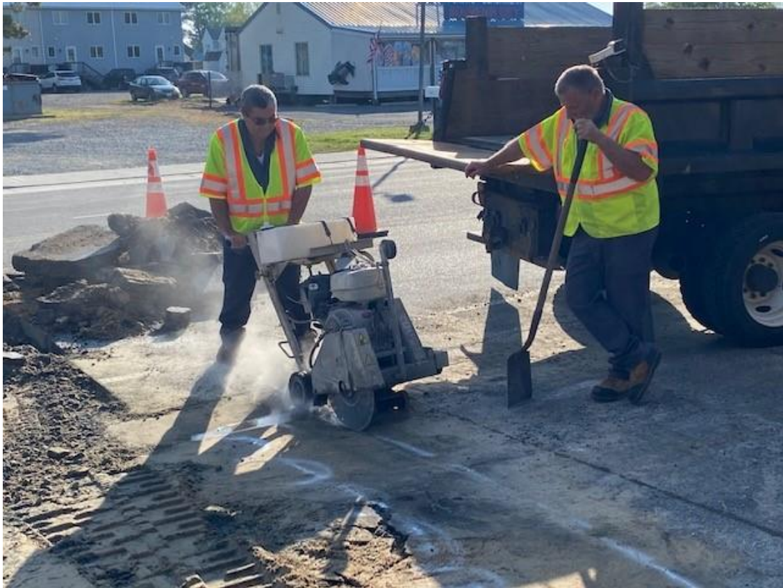
Saw cutting the damaged pavement
