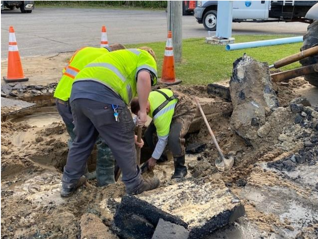
Excavating the damaged pipe
